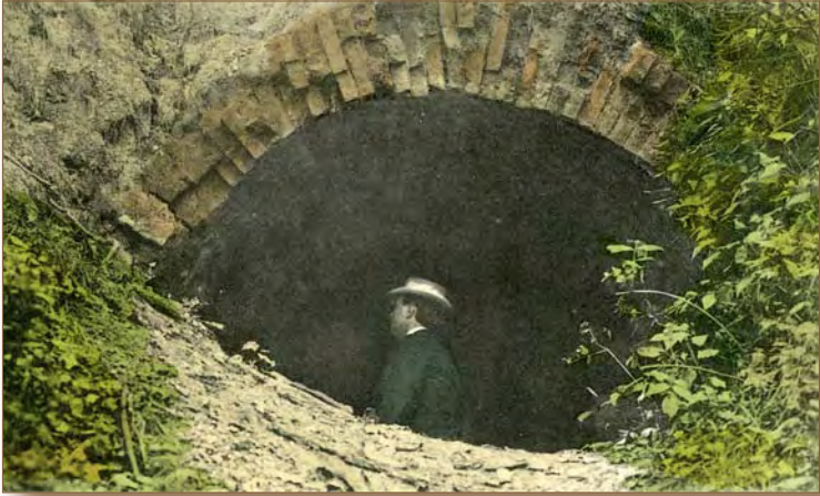
Tunnel entrance from Crosswicks Creek.
